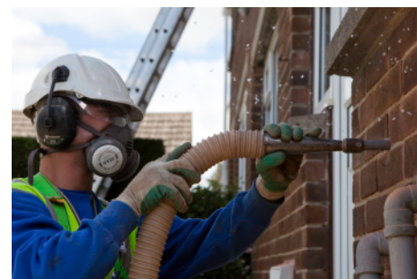
Installing cavity wall insulation in Kirklees, Yorkshire.
